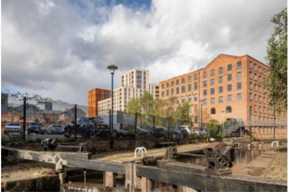
View P: Existing
